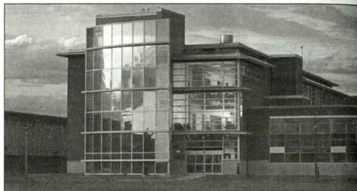
The Massachusetts Maritime Academy's new Storer Building in Bourne contains not only elements that call to mind ships and the nearby ocean, it also has been designed to safely ride out the worst onslaught that raging seas can create in the storm-surge flood zone in which it is located.
